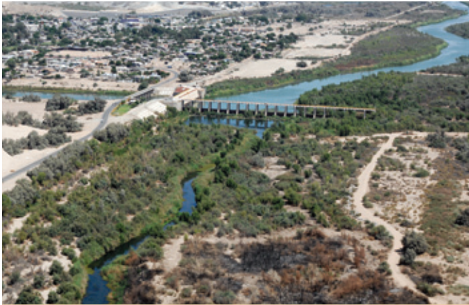
Morelos Dam Downstream View
