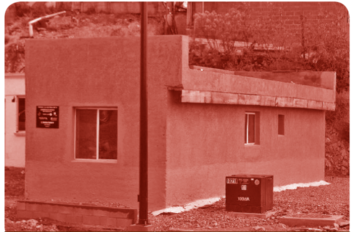
Completed Alcatel Lucent fibrous concrete house, Nogales, Sonora.
