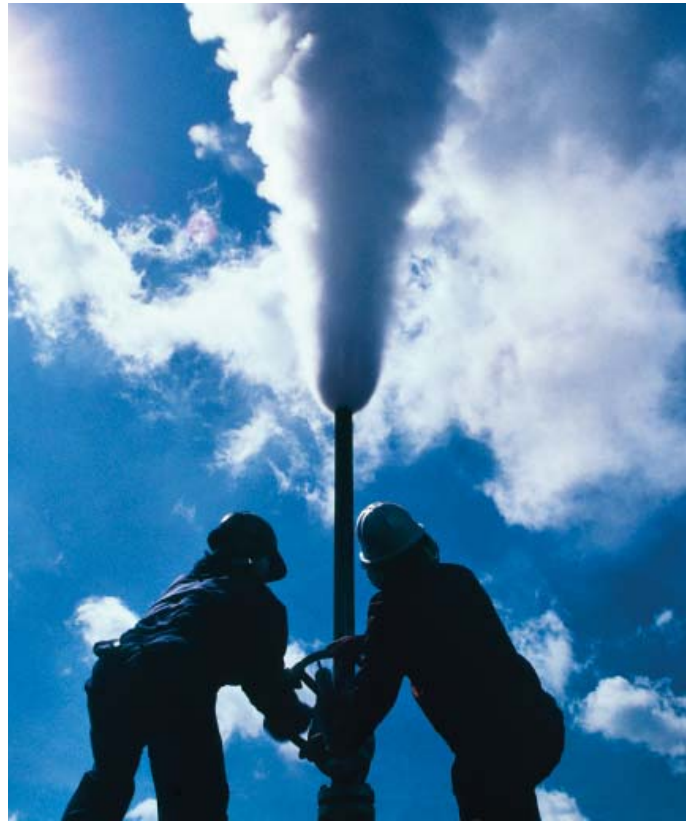
Geothermal pipeline being vented. ©Mayumi TeraoliStockphoto
