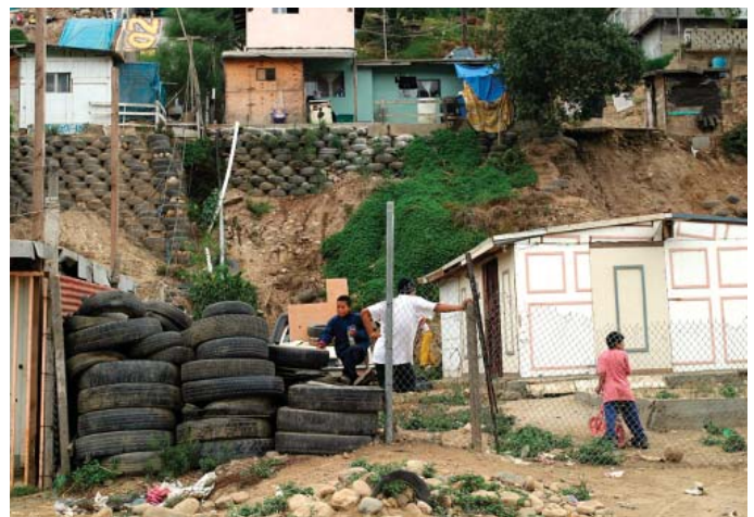
Scrap tires used as foundations for informal housing, Los Laureles Canyon, Tijuana. ©Paul Ganster
