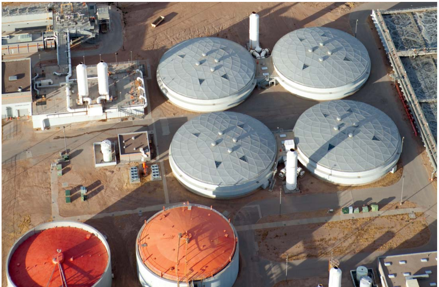
Wastewater treatment plant in El Paso, Texas. ©Krista Schlyer
