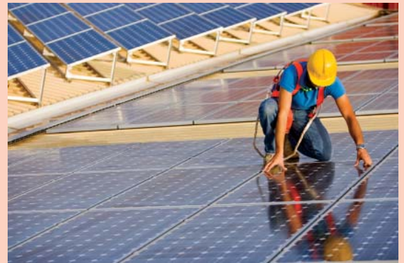
Worker inspecting a photovoltaic installation. ©Pedro CastellanolStockphoto
