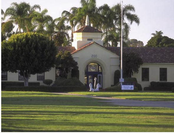
The historic buildings at the former Naval Training Center in San Diego are being restored and reused.
