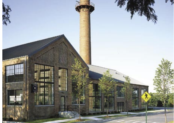
Modern updates to historic buildings make office space in Watertown Arsenal enticing.
