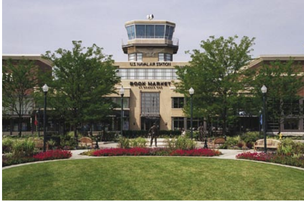
The former control tower was converted into a bookstore at Glenview Naval Air Station.
