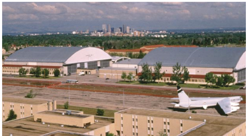
The conditions at Lowry Air Force Base before redevelopment.
