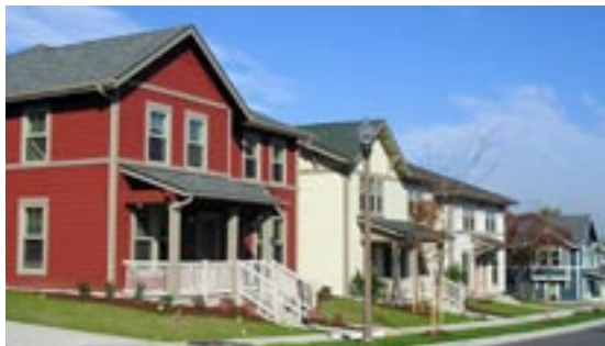
The design of Salishan redevelopment reduces impervious surface area, allows treatment of runoff on site, and restores and enhances wetlands with pedestrian paths—all while meeting density goals.
