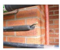
A Schrader badly fitted into the end of a poorly sealed copper pipe
