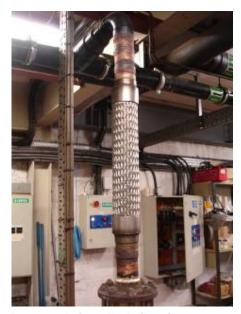
Incorrectly installed vibration eliminator
