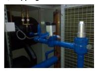
Capped stop valve to the right of the photo with the control actuator to the left
