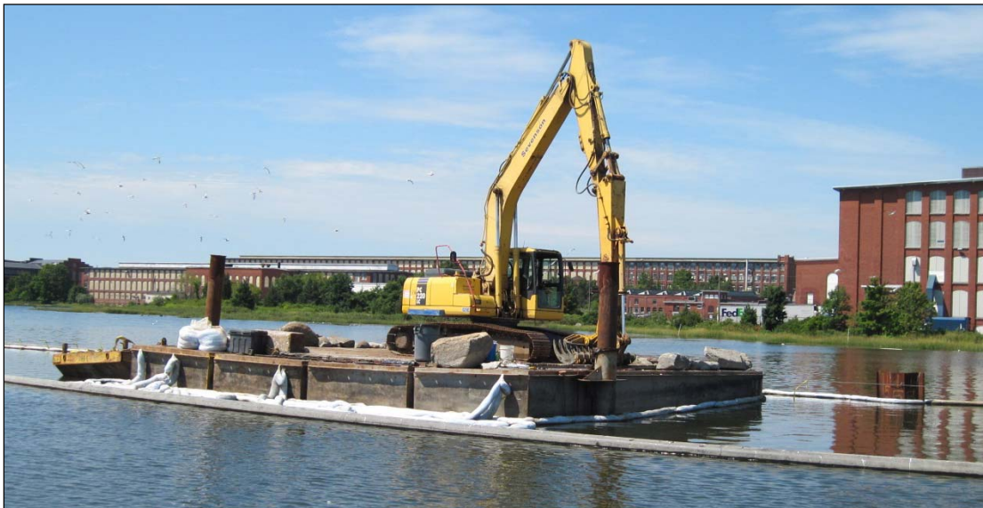
Figure 7. Debris Removal Excavator and Debris Storage Scow
