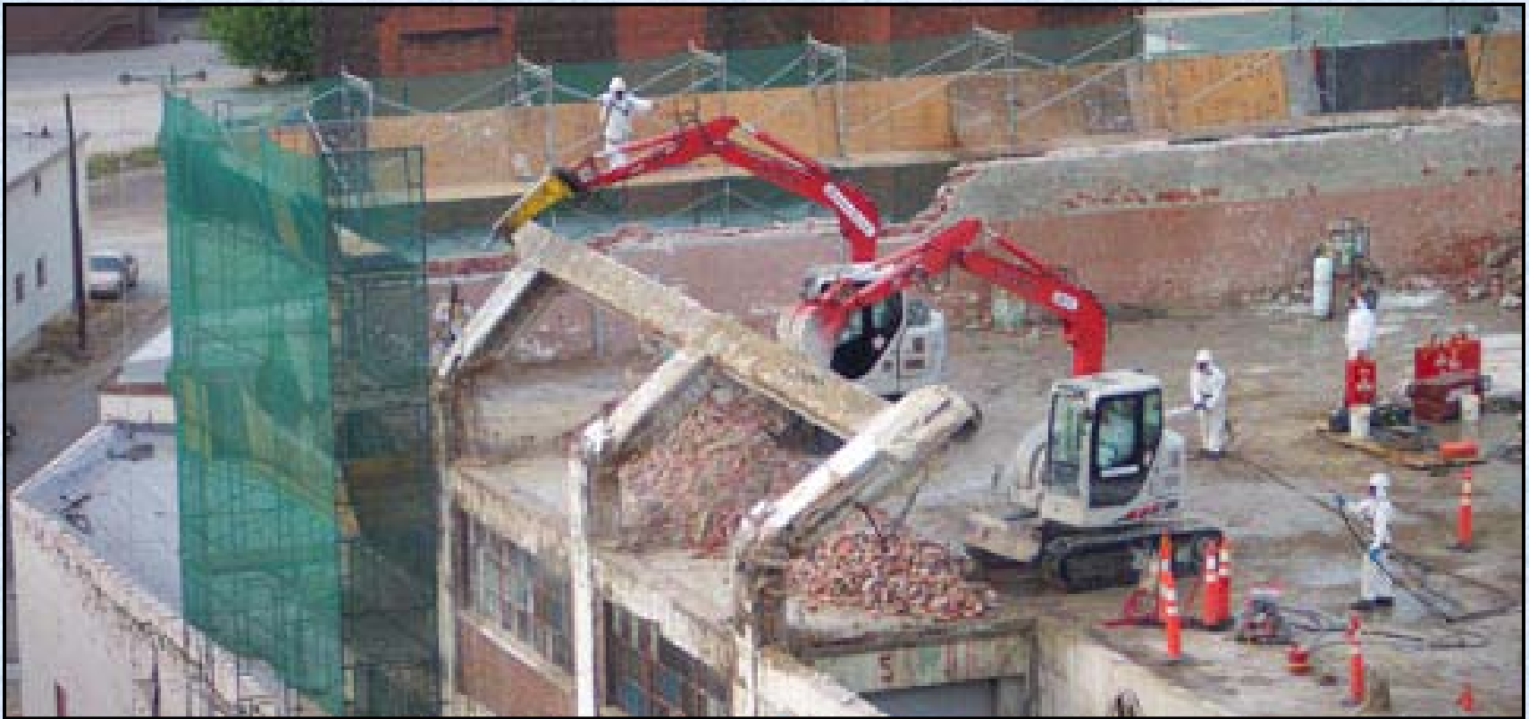
Demolition in Progress
