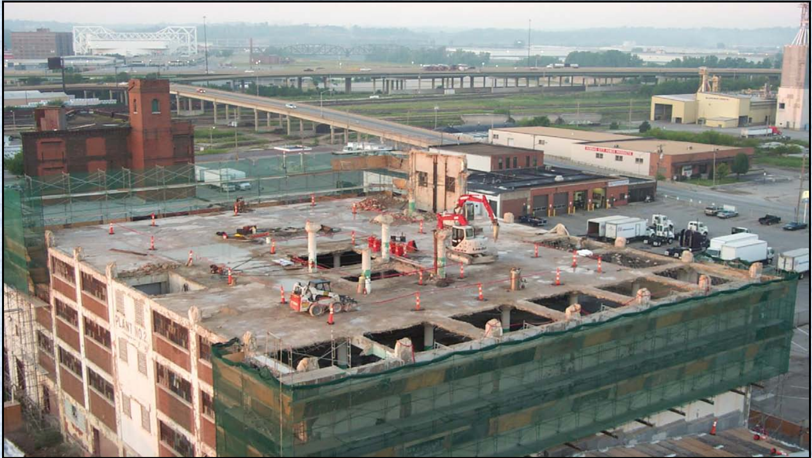
Demolition in Progress
