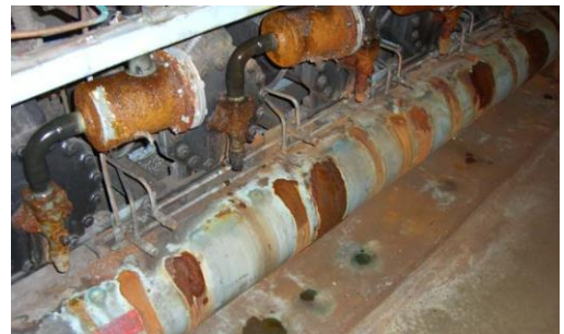
Excessive corrosion on rack components
