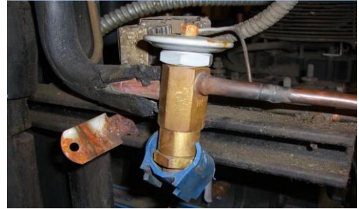
Image of broken clamp caused by vibrations
