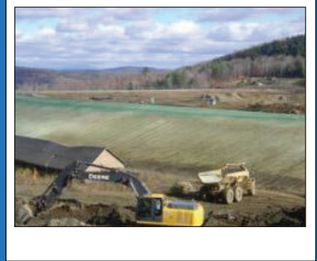
Elizabeth Mine stream and river restoration.
