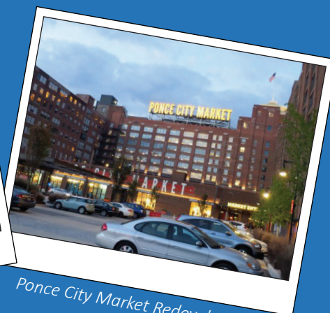
Former Sears Roebuck Warehouse.
