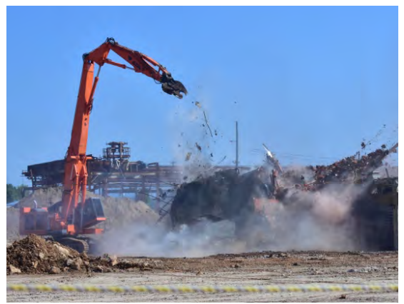
Building K-27, before and during demolition, 2016.
