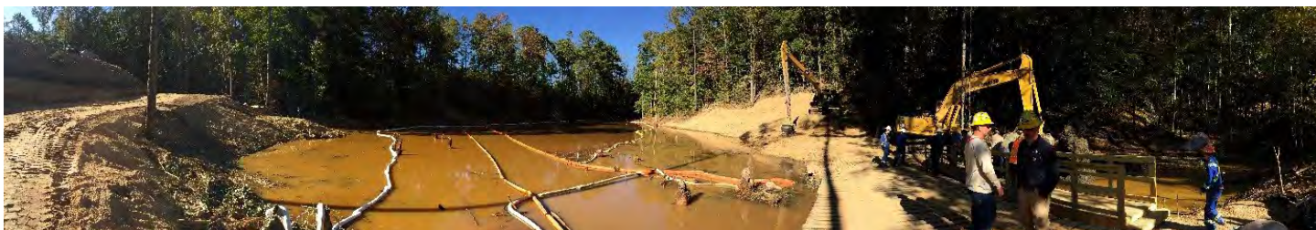
The pond after removal of gasoline and shoreline excavation.
