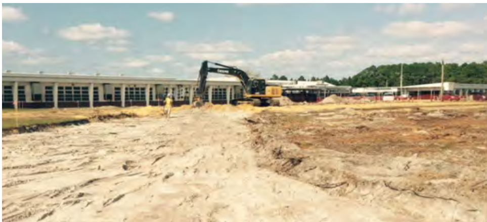
Excavation underway at Tyndall Elementary School.
