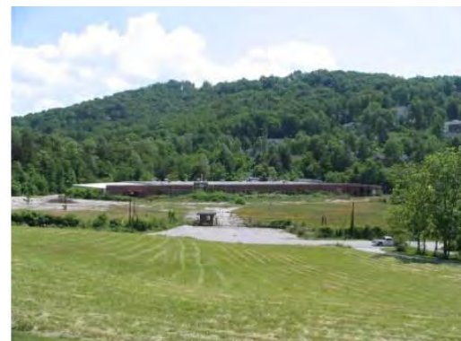
View of the CTS of Asheville, Inc. site.
