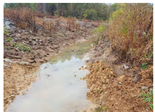
Top: View of the site's containment cell. Bottom: Hughes Creek following cleanup, November 2016.
