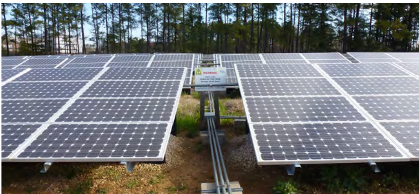
Solar panels on the capped part of the site.
