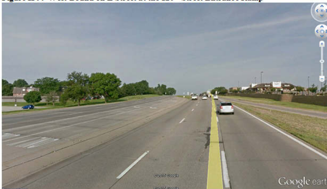
Figure H-9: West-Bound on L Street at the 120 th Street Entrance Ramp
