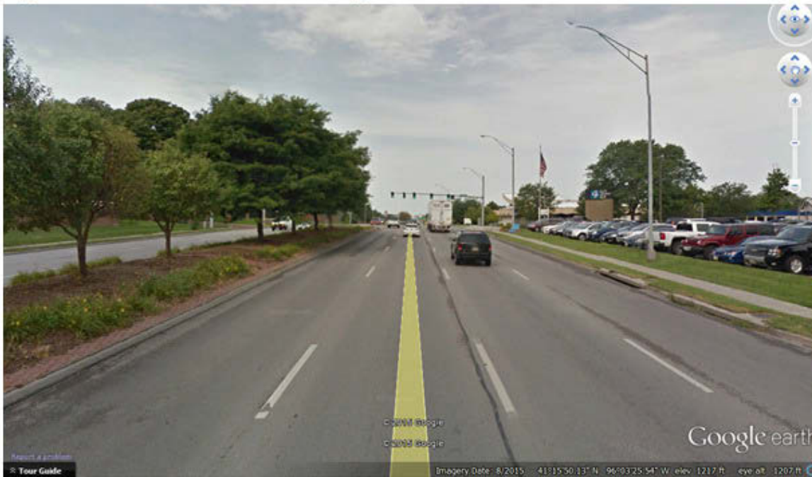
Figure H-7: West-Bound on West Dodge Road between 90 th and 93 rd Streets
