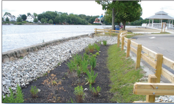
Figure 2. Rain Garden 1 (approximately 600 ft 2 ) collects and treats stormwater runoff from 11,270 ft 2 of Sunset Lake beachfront parking lot.
