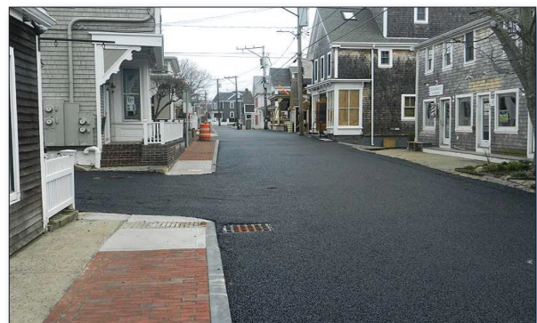
Figure 1. Porous pavement installation on Commercial Street, during (top) and after (bottom) construction.
