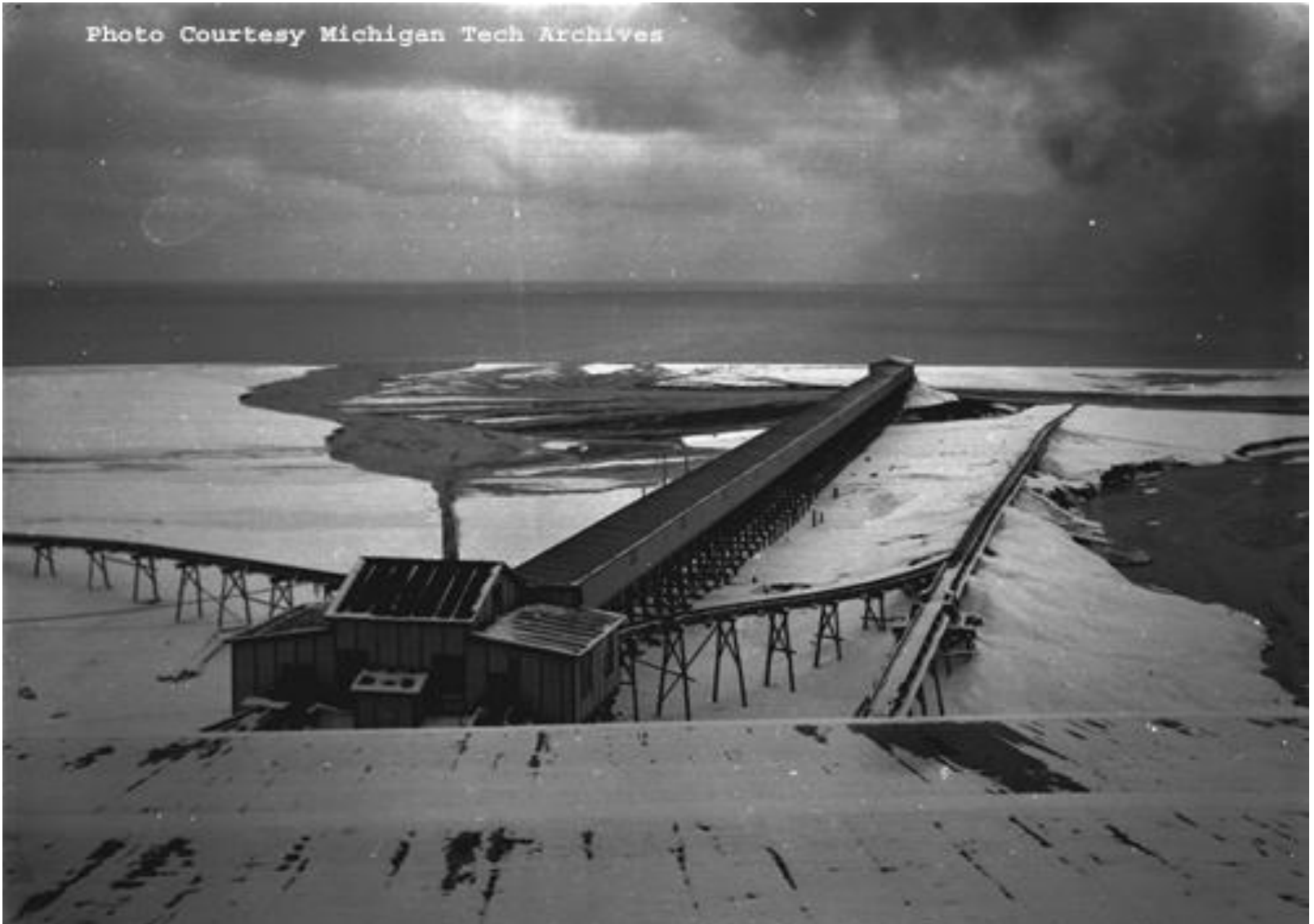
Fig. 5b. Primary and secondary sluiceways (Wolverine Mill, winter 1922?) carry stamp sands over the Gay pile. Lake Superior is on the horizon. Notice melted regions with fresh discharges.
