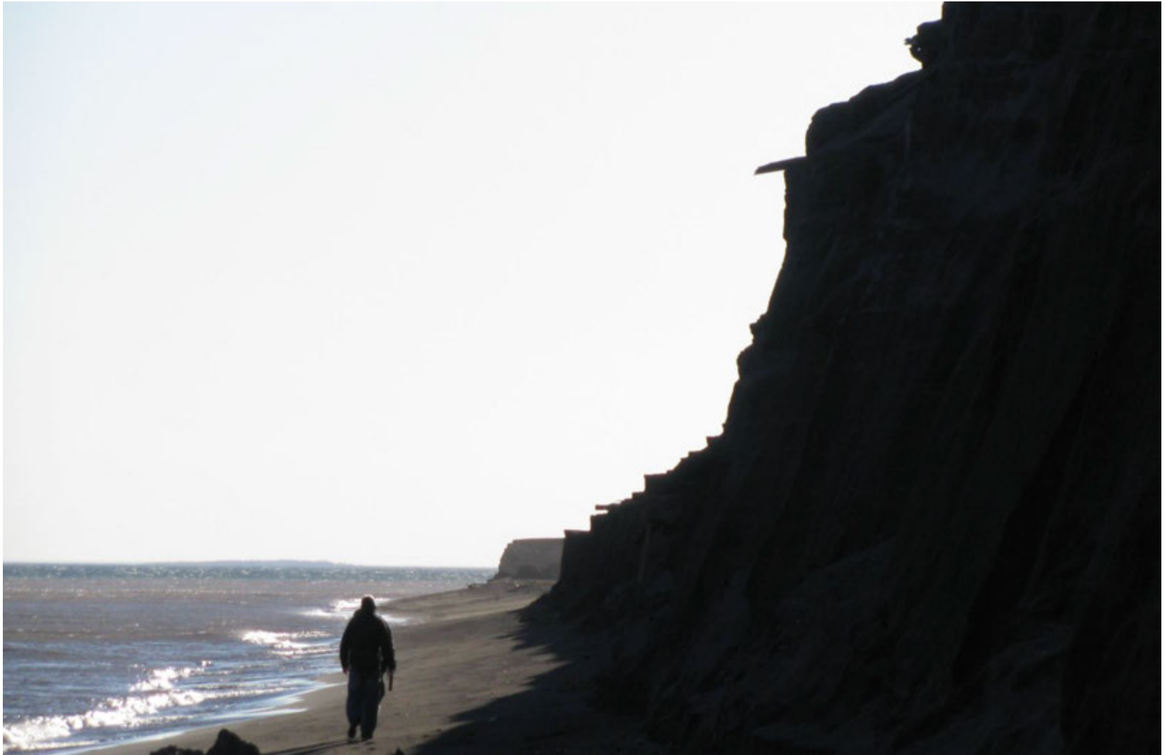
Figure 5a. Wave erosion of the Gay tailings pile. The near-vertical 7 m bluffs contain well-preserved remnants of wooden troughs that sluiced stamp sands across the pile.
