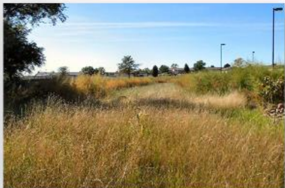
Vegetative swale Fort Carson, CO
