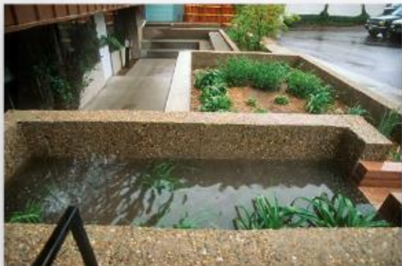
Rainwater collected in planter box then channeled into rain garden Boulder, CO
