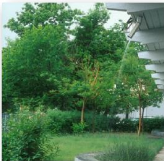
Irrigation by disconnected downspout Denver, CO
