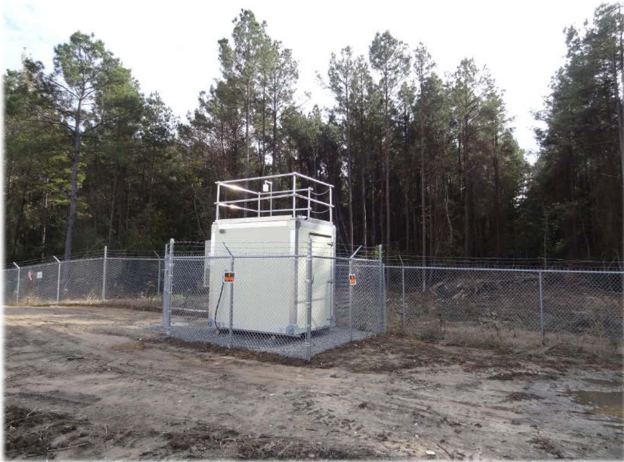
Hydrogen sulfide monitoring equipment in Crossett
