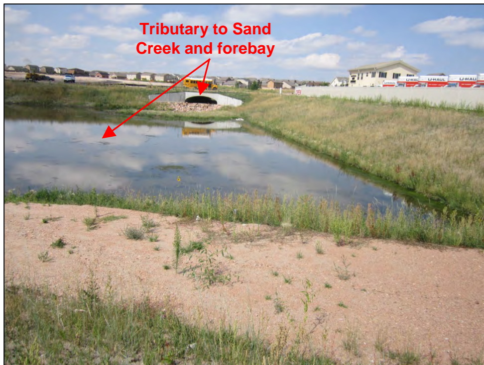
Photograph 134. View of what appeared to be a tributary of Sand Creek and one of two constructed forebays.
