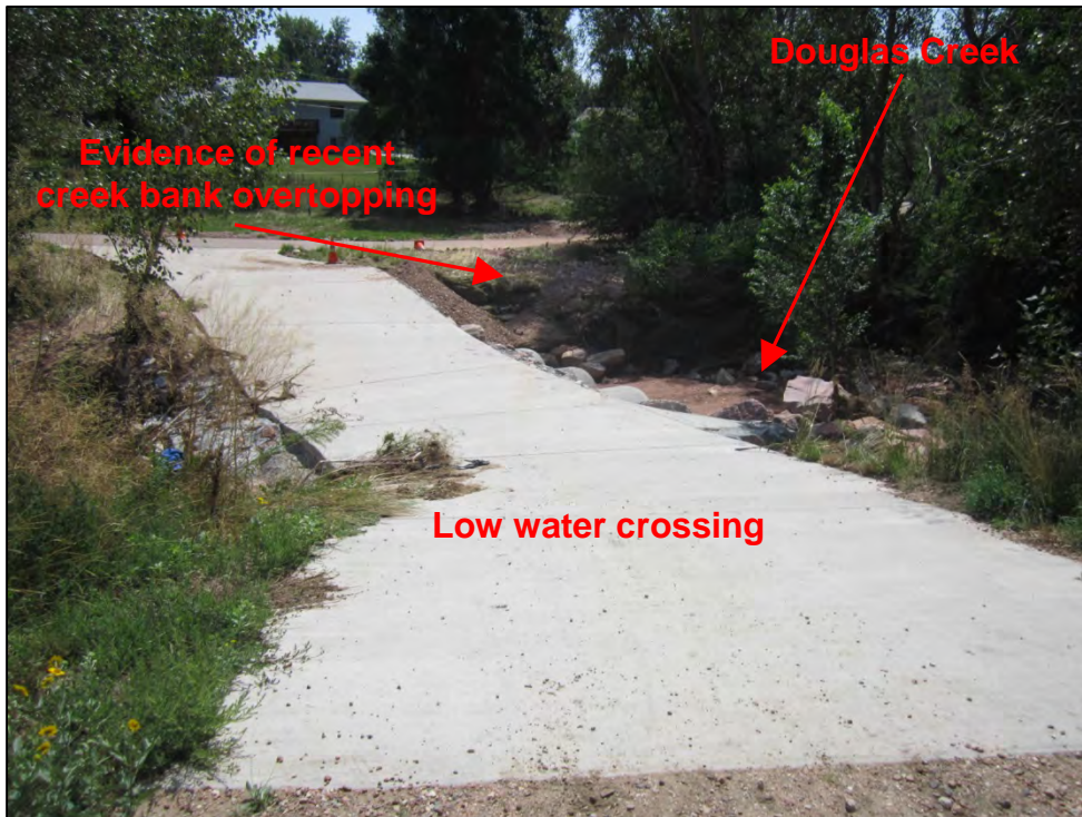
Photograph 18. View of CS – 016 Location No. 2 in-stream low water crossing (Texas Crossing).
