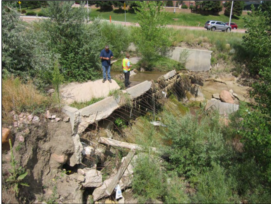
View of CS – 222, Rockrimmon Channel concrete drop structure.
