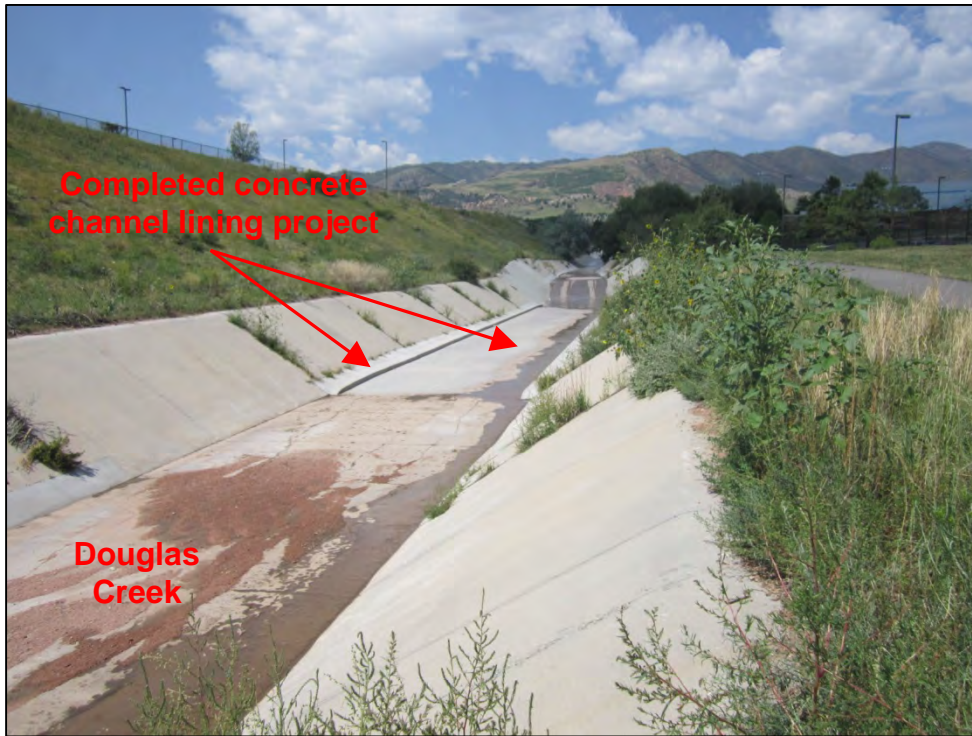
Photograph 17. View, facing upstream, of CS – 016 Location No. 1 completed concrete channel lining project on Douglas Creek near Intel Way.
