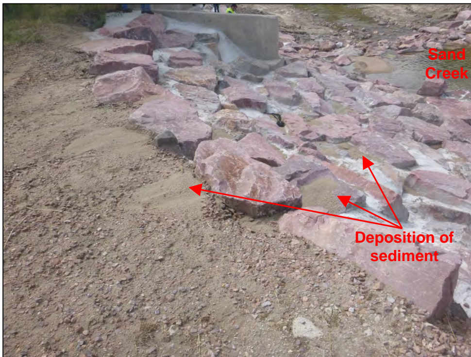
Photograph 100. View, facing downgradient, of the release of sediment across the sidewalk, shown in Photograph 99. Note the evidence of the previous release of sediment and deposition of sediment into Sand Creek.
