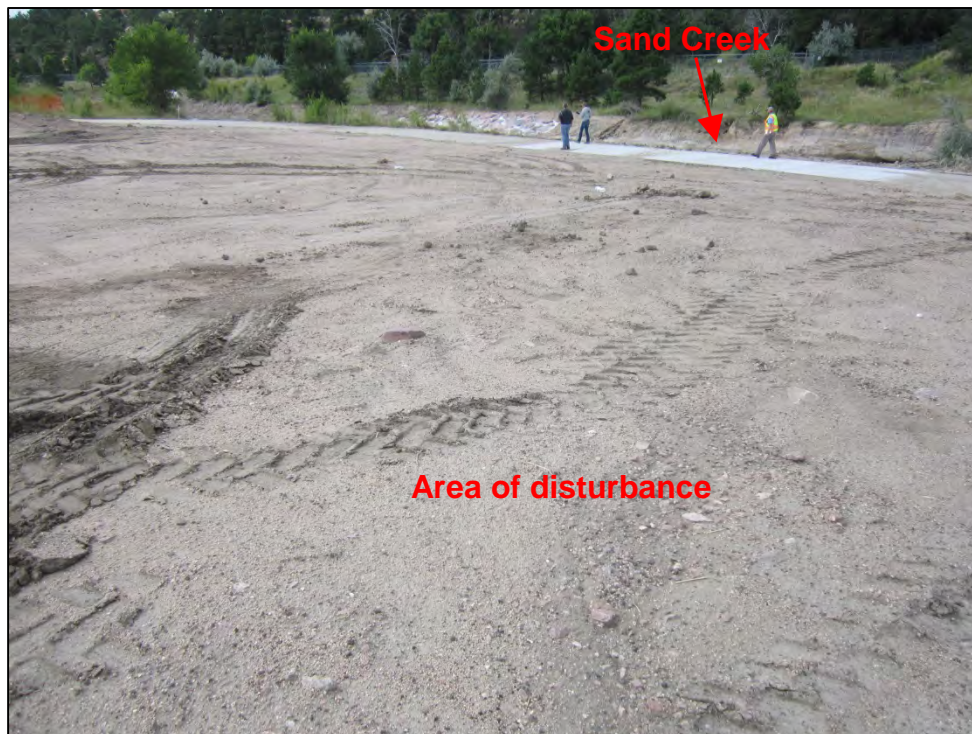
Photograph 96. View of the denuded area of disturbance utilized by the City's contractor as a staging area for the in-stream Sand Creek project located near 1355 Space Center Drive. Note the lack of erosion, sediment, and perimeter controls.
