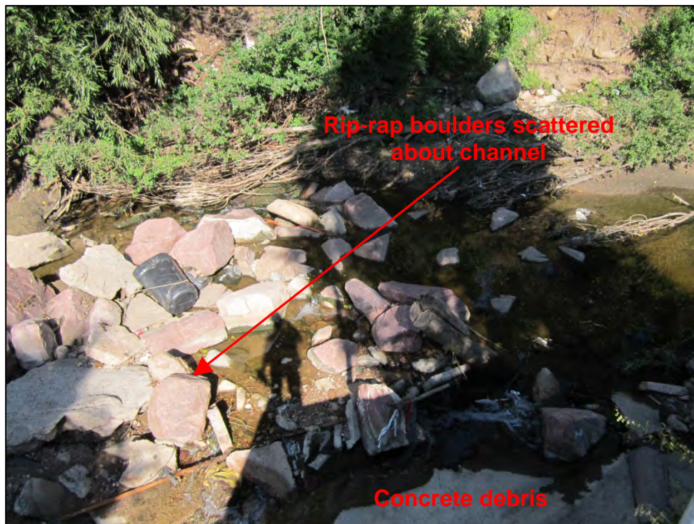
Photograph 4. Close-up view of the rip-rap boulders, concrete debris, and waste scattered throughout the Shooks Run channel near the confluence with Fountain Creek, shown in Photographs 2 and 3 above.
