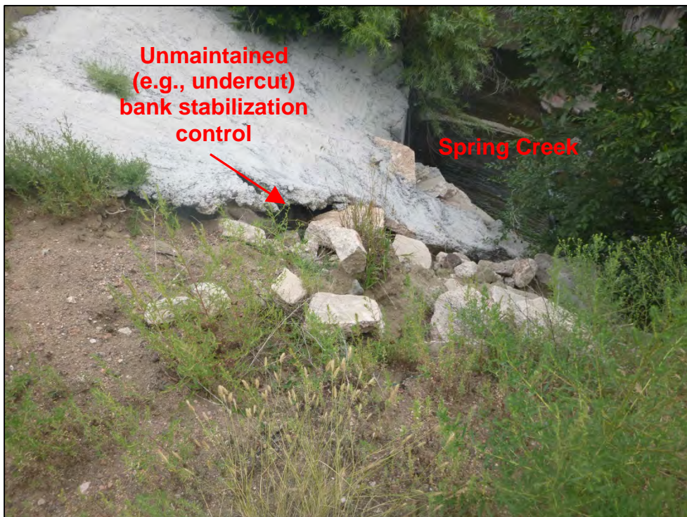
Photograph 88. View of CS – 362 Spring Creek near 3667 E. Bijou Street. Note the unmaintained (e.g., undercut) Spring Creek box culvert bank stabilization control.
