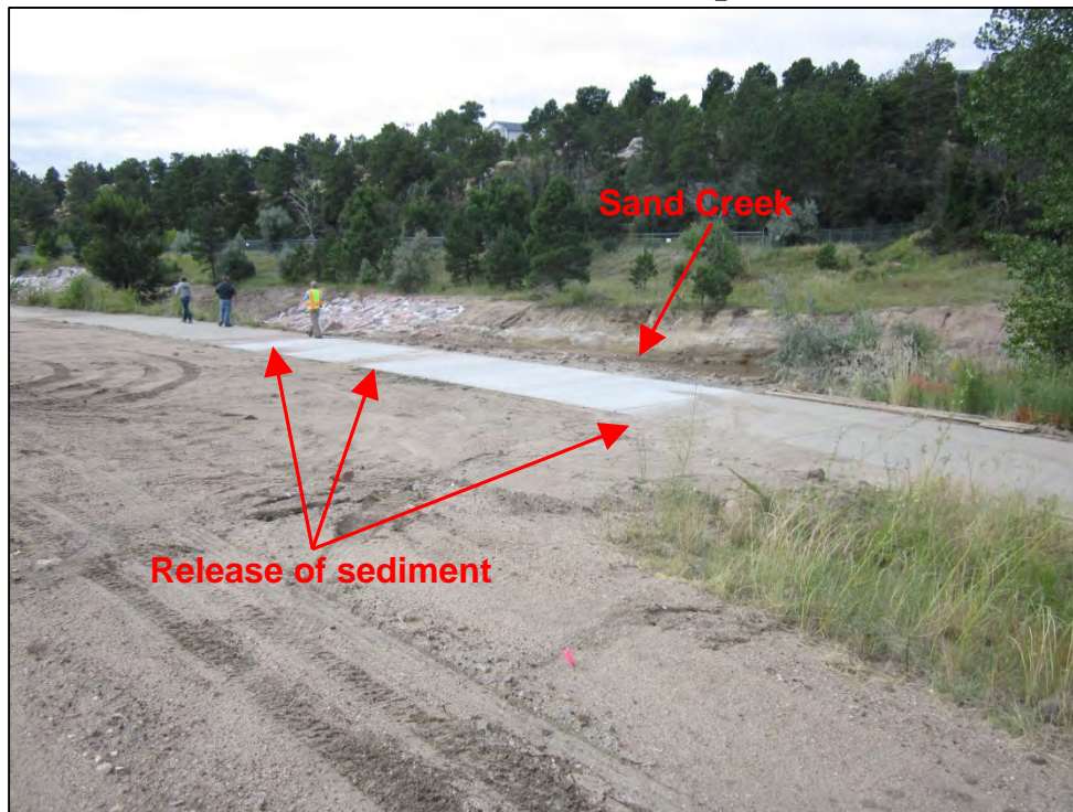
Photograph 97. View of evidence of previous erosion and the release of sediment across the sidewalk toward Sand Creek from the area of disturbance at the staging area, shown in Photograph 96.
