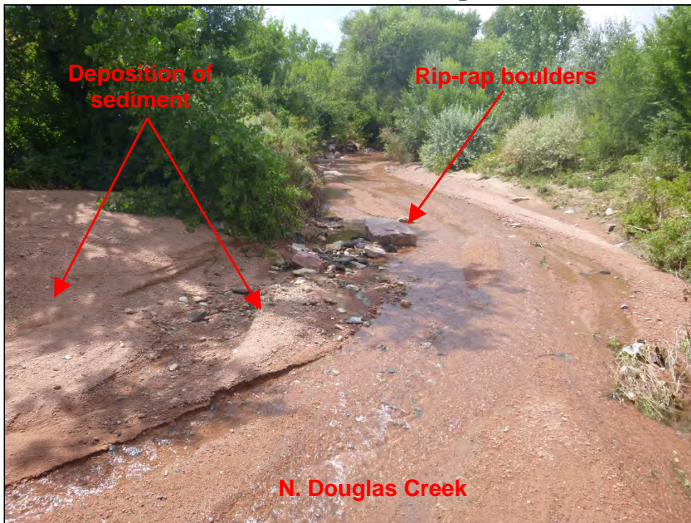
Photograph 39. View of deposition of sediment and rip-rap boulders in the N. Douglas Creek channel.
