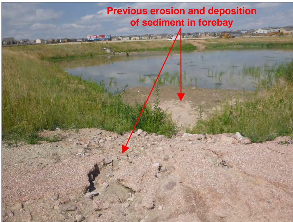
Photograph 137. View of evidence of previous erosion and deposition of sediment in forebay, shown in Photograph 135 and 136.
