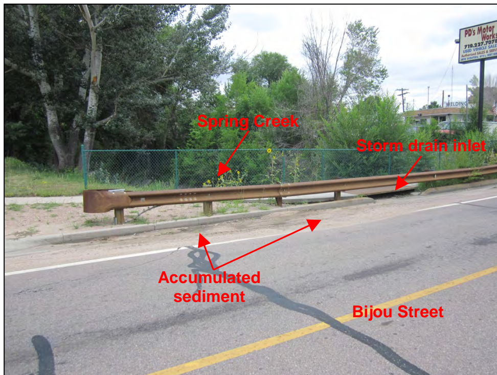
Photograph 90. View of accumulated sediment on the roadway and adjacent to the storm drain inlet on the other side of Bijou Street, shown in Photograph 89. Note that this storm drain inlet also drains directly to Spring Creek.
