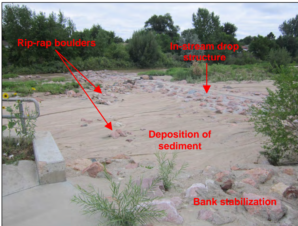
Photograph 80. View of Sand Creek just upstream of MS4 conveyance channel (shown above) outfall. Note the deposition of sediment and rip-rap boulders scattered about Sand Creek in the vicinity of a constructed in-stream drop structure.
