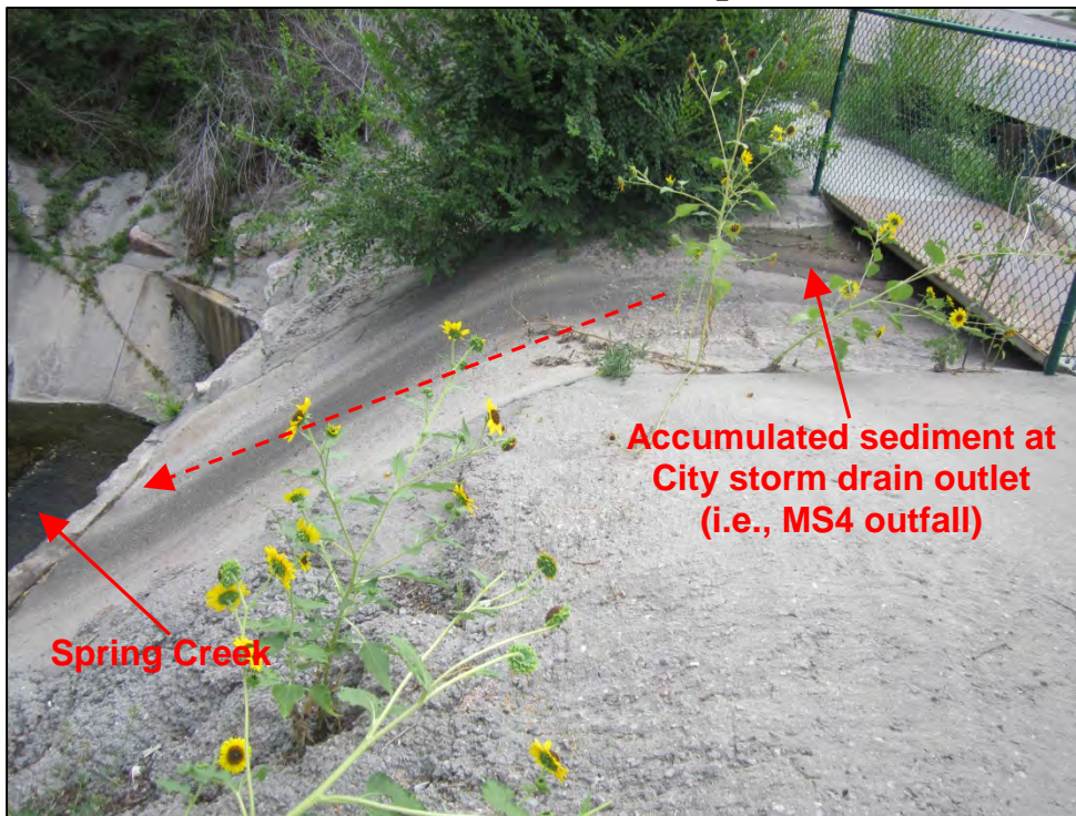
Photograph 91. View of accumulated sediment at City storm drain outlet (i.e., MS4 outfall) shown in Photograph 90.
