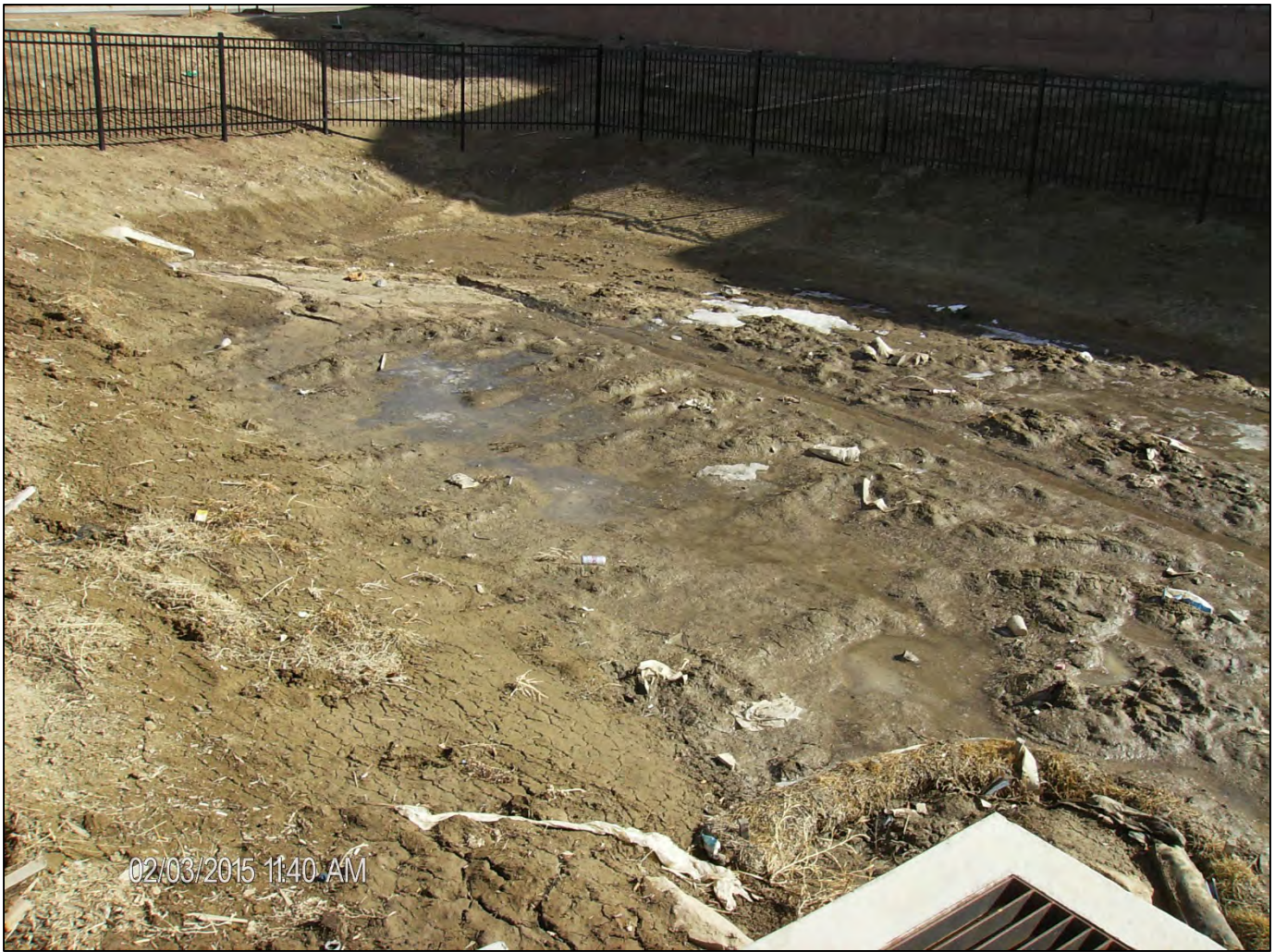
Exhibit 21. City provided photograph of ID – 070 Woodmen Ridge Apartments EDB, dated February 3, 2105. Note that the EDB was unstabilized and contained accumulated sediment and debris.
