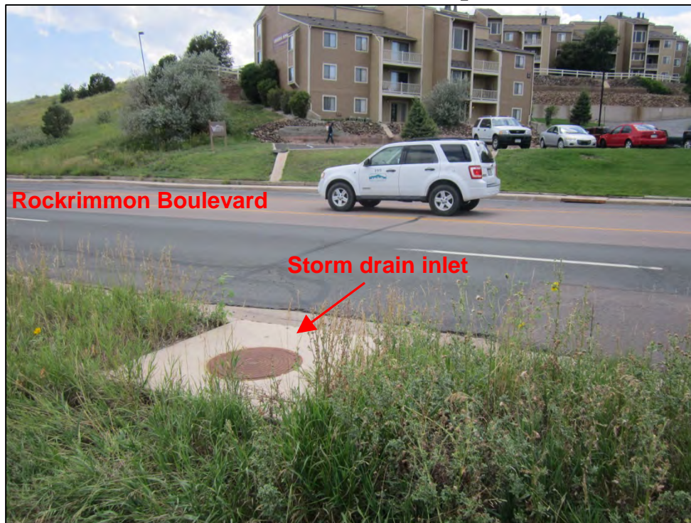
Photograph 43. View of CS – 015 storm drain inlet on Rockrimmon Boulevard. Note that the upgradient drainage areas from private residential development areas and City streets appeared to lack source control BMPs for flow attenuation.
