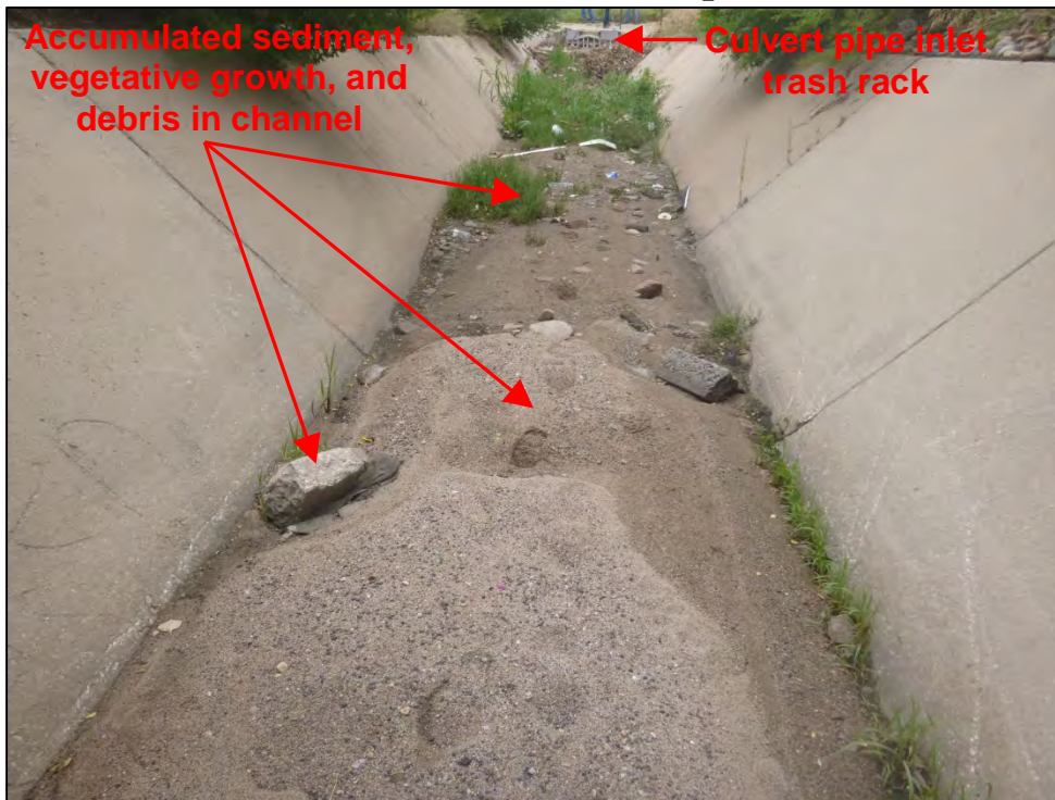
Photograph 67. View, facing downstream, in channel of accumulated sediment, vegetative growth, and debris within the concrete lined channel located just upstream of the culvert pipe inlet trash rack, shown in Photograph 66.
