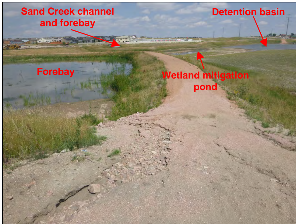
Photograph 133. View of Forest Meadows Drive and Vollmer Drive – Detention/Wetland Mitigation. Note the location of the Sand Creek channel, two forebays, wetland pond, and main detention basin.
