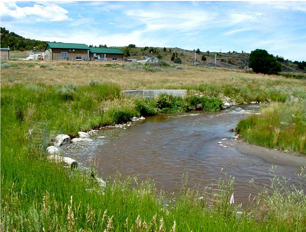
Figure 3 - Discharge Point 002A into Rock Creek
