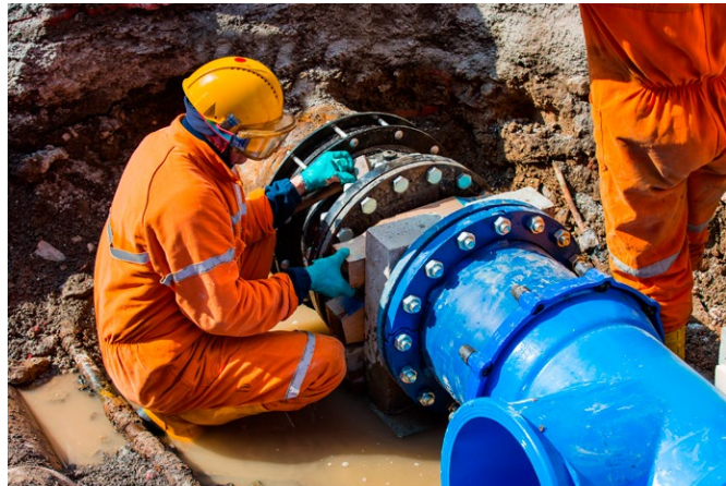
Water infrastructure construction for new development. Credit: Muratart / Shutterstock.com.
