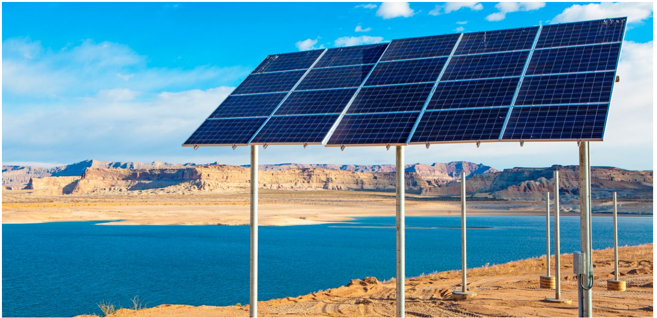
Solar panels along the shore of Lake Powell. Credit: Susan Schmitz / Shutterstock.com.
