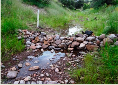
A rock erosion-control structure provides a localized increase in water infiltration in the Chiricahua Mountains. Credit: Sky Island Alliance.
