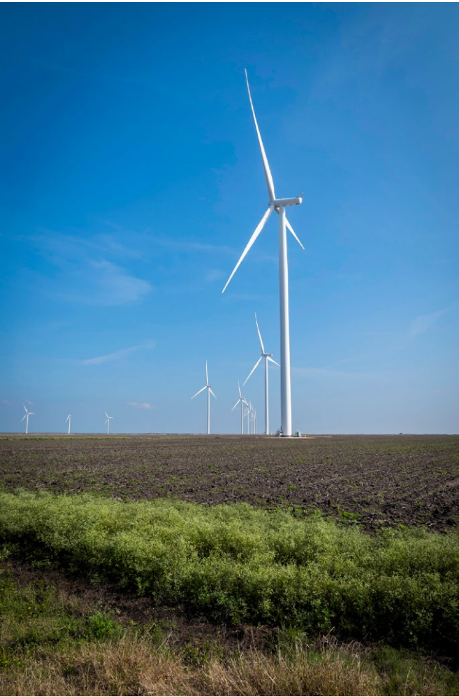
The 200-megawatt Los Vientos I Windpower Project is in Lyford, Willacy County, Texas. Together with its sister project Los Vientos II, it powers about 280,000 homes. Credit: Duke Energy Renewables.
