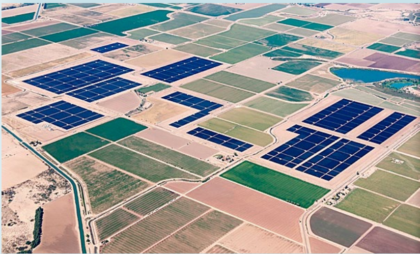
The Campo Verde Solar Facility (139-megawatt alternating current) is located in Imperial County, California, less than 10 miles from the U.S.-Mexico border.
