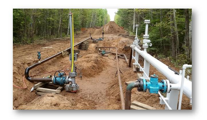
Smaller-diameter pipeline stopple bypass
