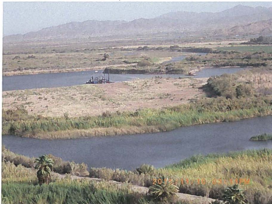
Close up view of the dredge working in Area C.
