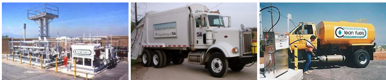
Figure 3-12. LNG Station and LNG-Powered Trucks
