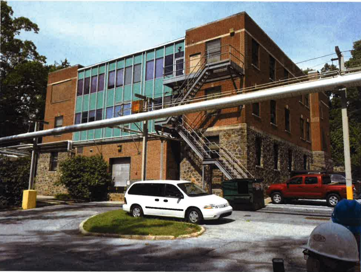
Photograph 7. Southeastern corner of Building 249 facing northwest.
