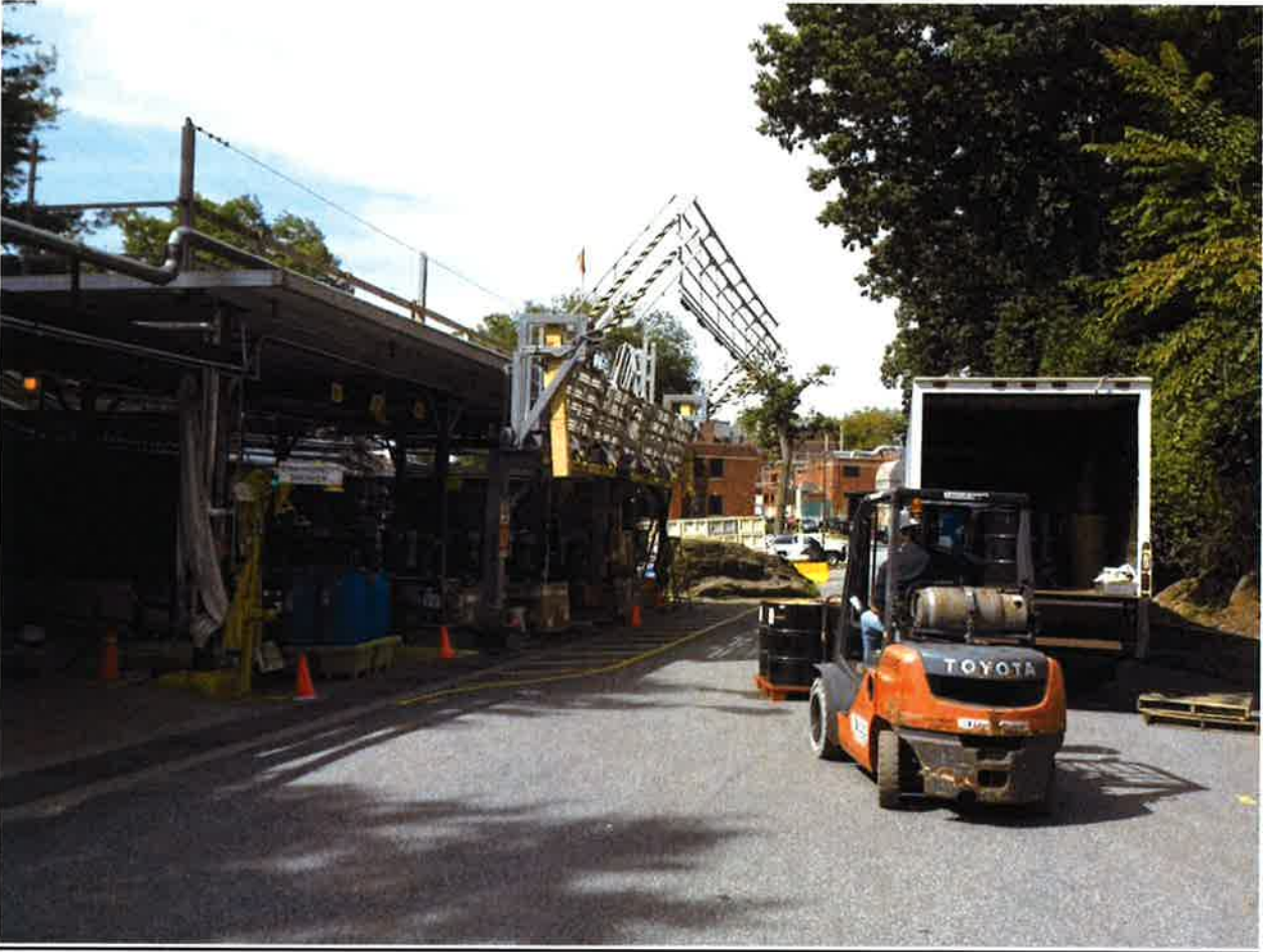
Photograph 1. Upper Creek Rd looking southwest.
