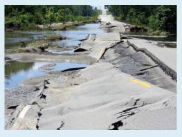
Flooding of the Cedar River in 2008 damaged this section of U.S. Highway 6 east of Atalissa. Credit: lowa Department of Transportation.
