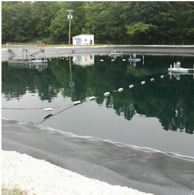
Picture 7: Wilcox WWTP
