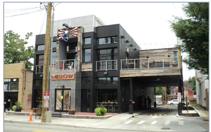
The newly constructed Mellow Mushroom Pizza Bakers restaurant.
