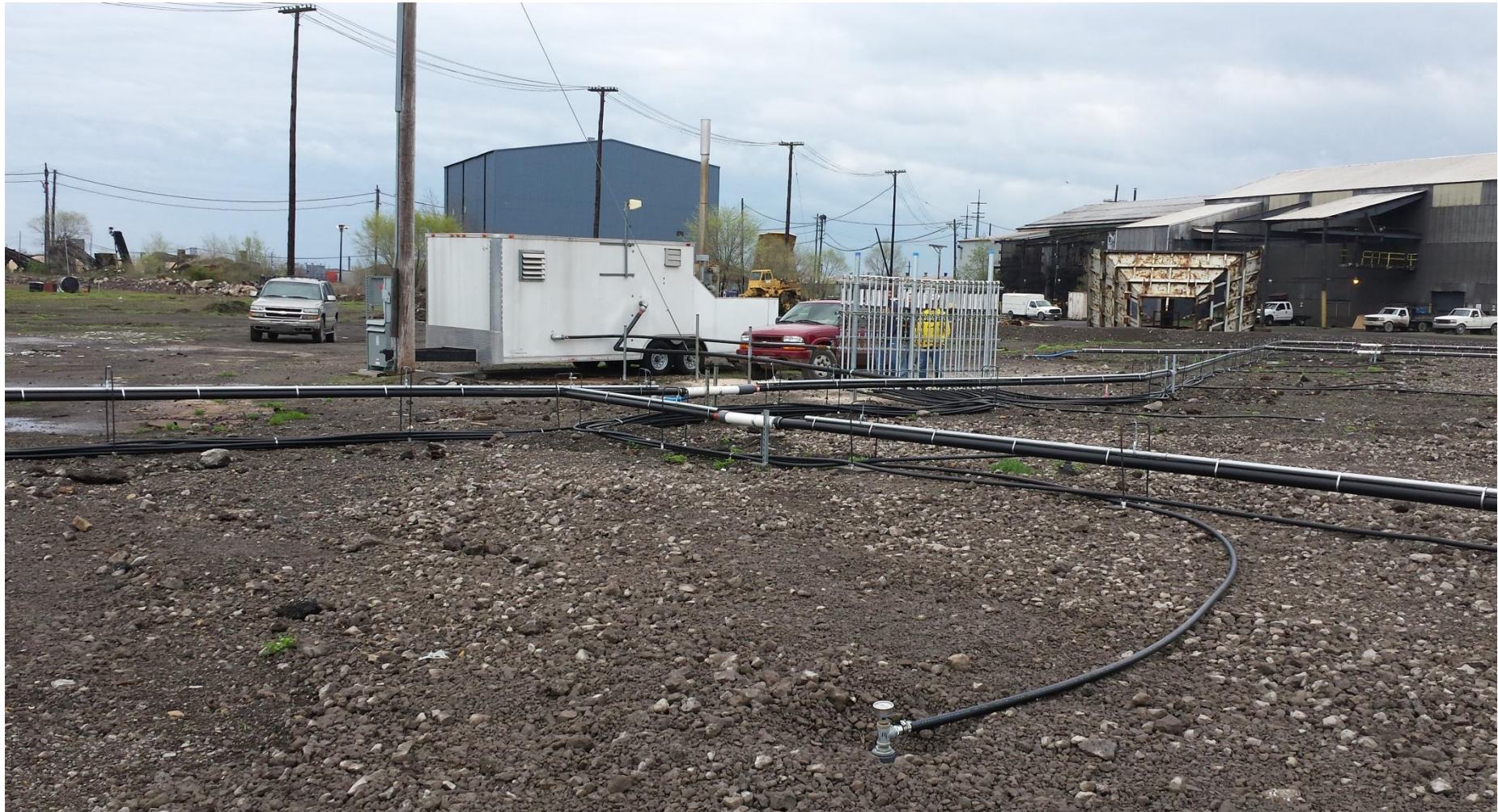
Cell 1 Piping System Completely Replaced and New Sparge Wells Added
