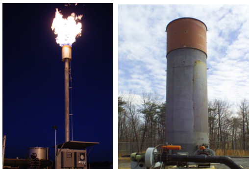
Figure 1-4. Open (left) and Enclosed (right) Flares
