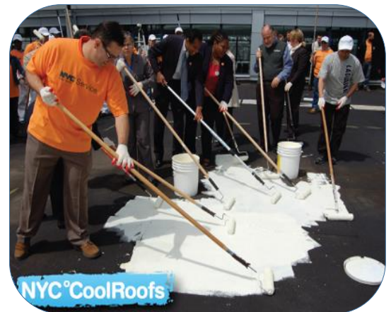
By painting roofs with white or reflective paint, New York City is reducing the urban heat island effect.
