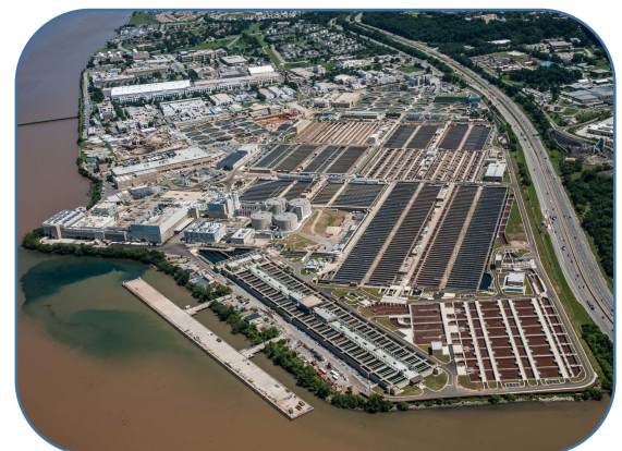
Future seawall at Washington, DC, Blue Plains Wastewater Facility will reduce the risks of flooding
