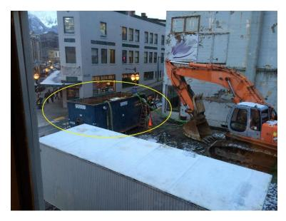
Figure 8. Water from a building demolition drained into the basement and was pumped to this tank (circled in picture) for settling before filtration to remove asbestos and other pollutants. Photo courtesy of John Pavitt, US EPA Region 10.
