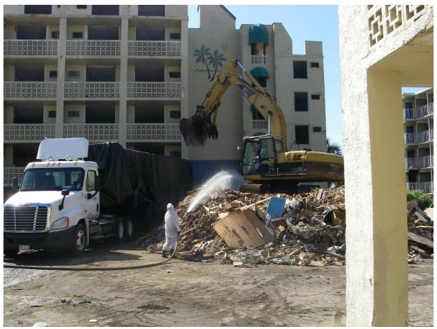
Figure 4. Ordered demolition of a structure on sandy soil in a coastal area. Water drains readily through this soil, and asbestos carried by the demolition water becomes embedded in the sandy soil. Photo courtesy of Pam McIlvaine, US EPA and Robin Mack, SCDEQ.
