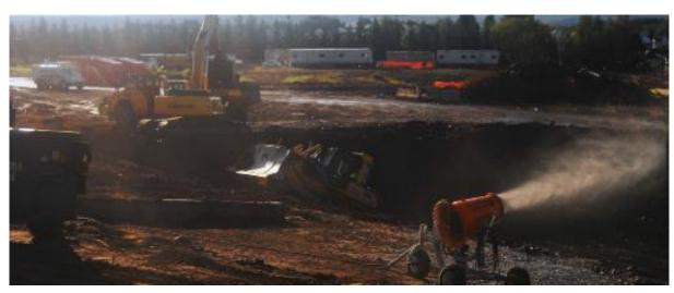
Figure 13. A machine delivering an atomized mist keeps materials adequately wet. This work is being conducted at a lead-remediation site with compliance requirements similar to the Asbestos NESHAP. (Photo used with permission from DustBoss, 2015). No endorsement is implied. Illustration provided for informational purposes only.
