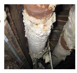
Figure 14. Pipe wrap is frequently hidden and may be difficult to find. Special wetting agents may be needed for pipe wrap.
