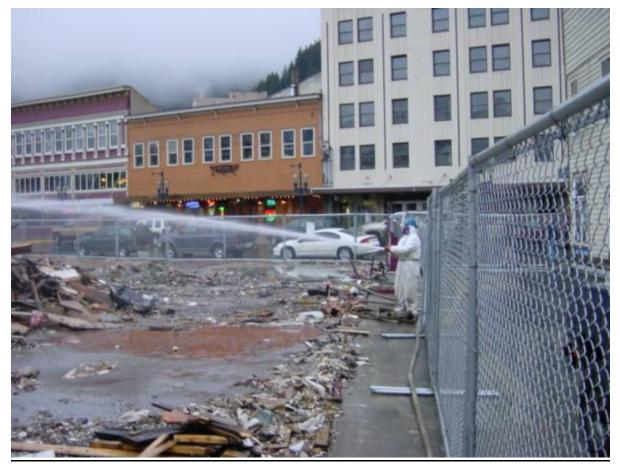
Figure 5. The surrounding sidewalk functions as a berm at this demolition, (EPA photo courtesy of John Pavitt, Region 10).
