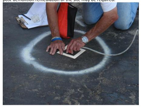
Figure 15. Micro-vac sampling is one method that may be used to indicate that non-porous surfaces, such as this asphalt parking lot, have not been contaminated by asbestos after the ordered demolition of the hotel featured in Figure 4. Photo courtesy of
