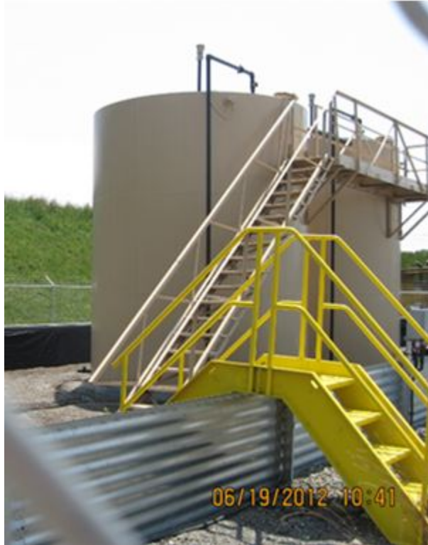
Figure B-12. Produced Water Storage Tanks
