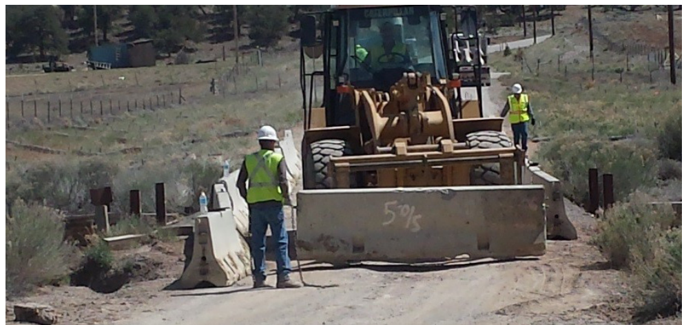
Safety barriers being placed along the community bridge.
