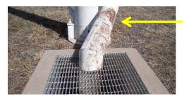
Overflows directly connected to a sanitary sewer or storm drain will trigger a significant deficiency; there must be an air gap of at least 3 pipe diameters above the sanitary sewer or storm drain. An air gap is needed to prevent a cross connection between the sewer or storm drain and the overflow pipe. This air gap also prevents the tank from inhaling air from a sewer or storm drain when the overflow is not spilling water, which should be most of the time.
