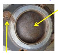
The #24 mesh screen can be installed between two flanges. After an overflow event the screen can be inspected and replaced, if needed.
