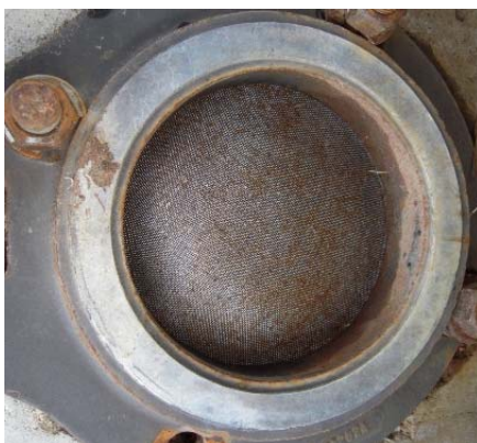
The best design is to install the #24 mesh screen between two flanges.
