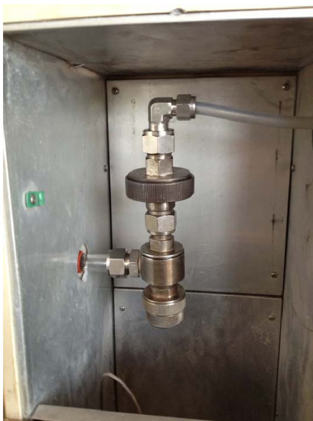
Figure 2-2. Heated Filter Box with PM 2.5 Cyclone and PM 2.5 Filter
