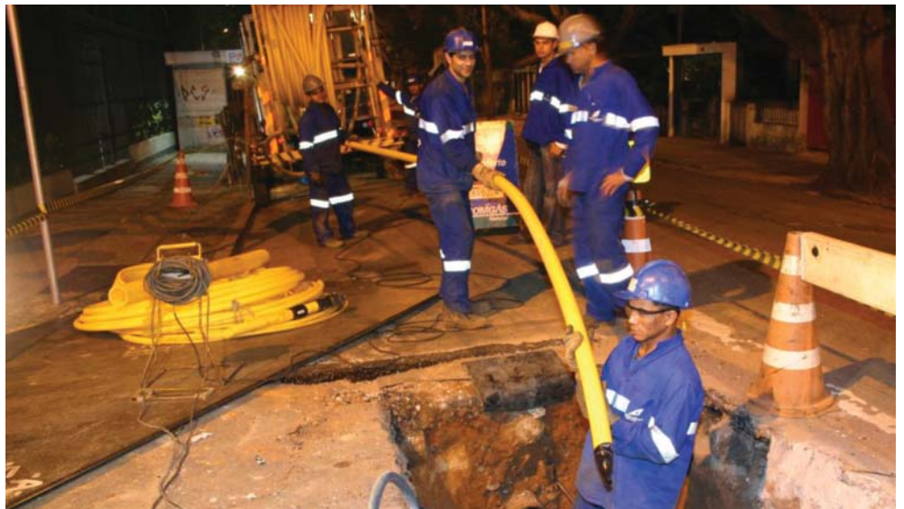
Polyethylene piping end ready to be inserted.
