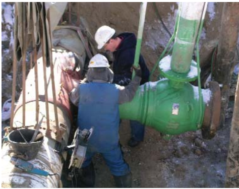
Employees of TransCanada work to update a natural gas line.
