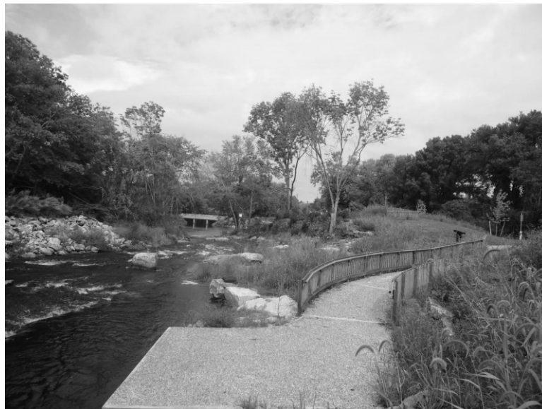
Photo: Richmond, RI ~ Knowles Mill
