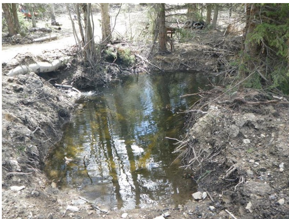
One of nine ponds illegally constructed on U.S. Forest Service land.
