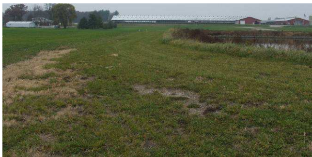
Location of W side TDLAS beam path, looking N towards the TDLAS/scanner system. Lagoon berm is on right
