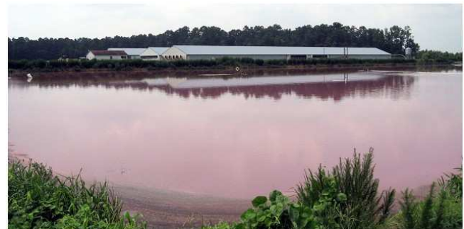
S berm looking from the NE berm corner.
