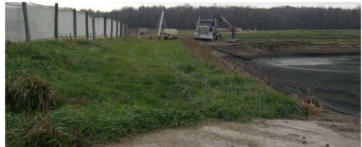
E side of lagoons looking S along W side of fenceline. 1 st stage lagoon is on right.
