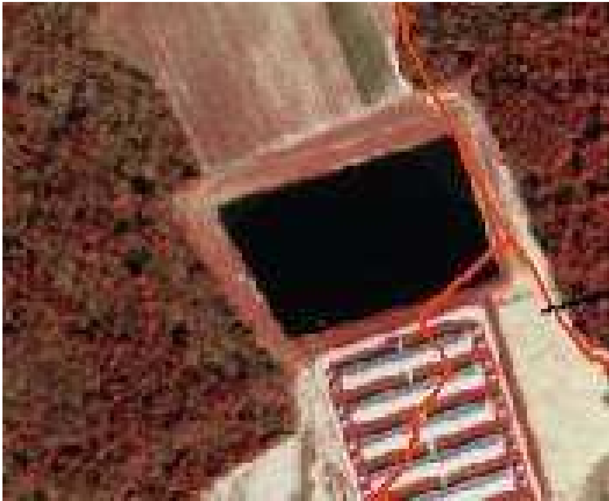
Figure 1. Aerial view of lagoon, showing relationship to the barns. Red lines indicate soils delineations, and not a physical property boundary.
