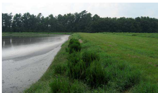
N berm looking W towards NW retro-reflector tower location.
