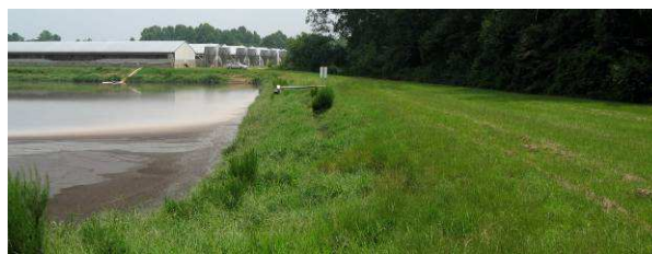
W berm looking S towards SE retro-reflector tower location.
