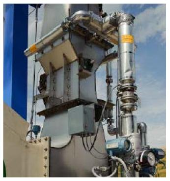
No Moving Internal Parts One Fan and One or Two Pumps High Alloy Parts Fabricated from Flat Stock
