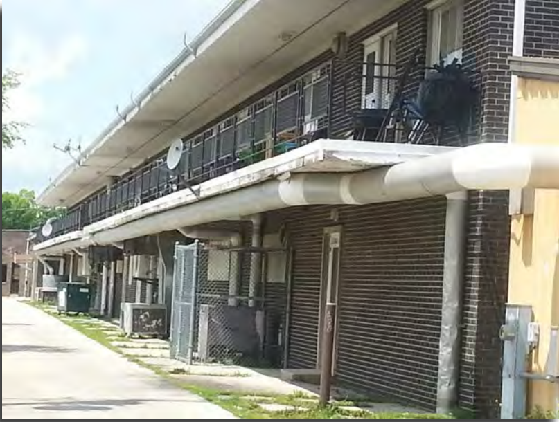
Building located next to Yeoman Creek Landfill which houses apartments and businesses.
