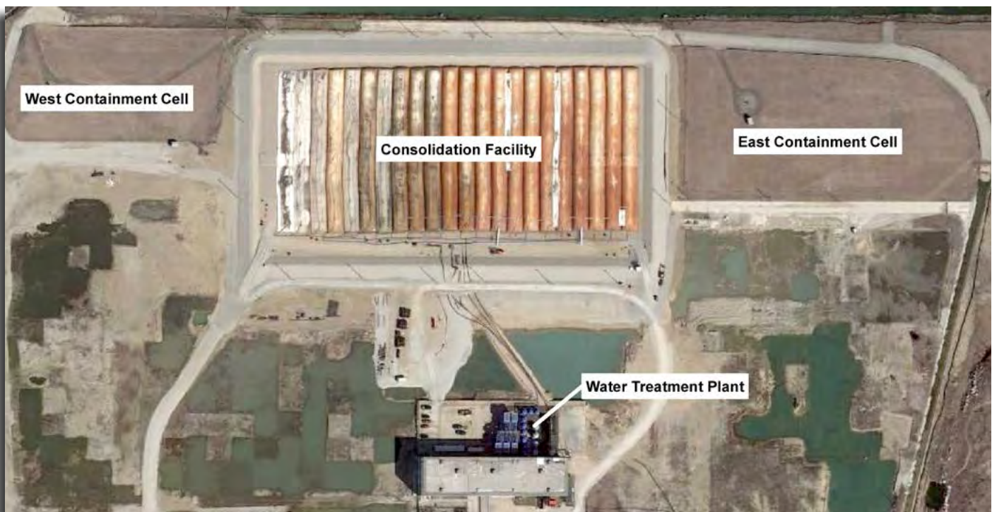
The containment cells and water treatment plant at OMC.
