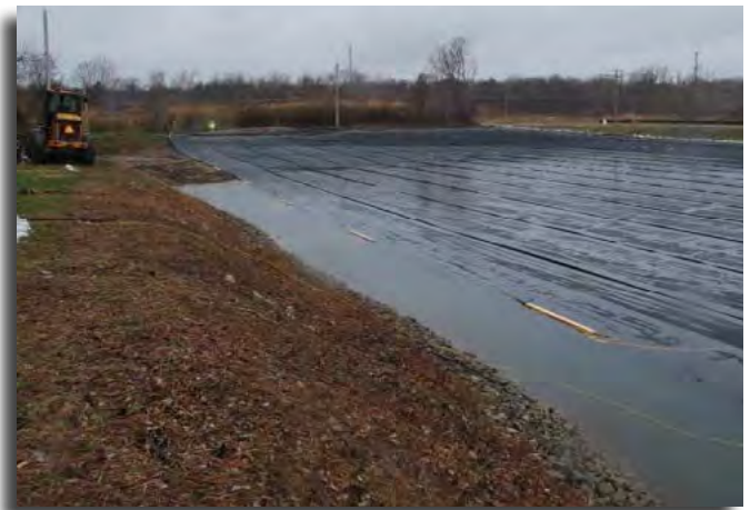
This photo shows the geotextile pull (80% complete) at the pumping lagoon.
