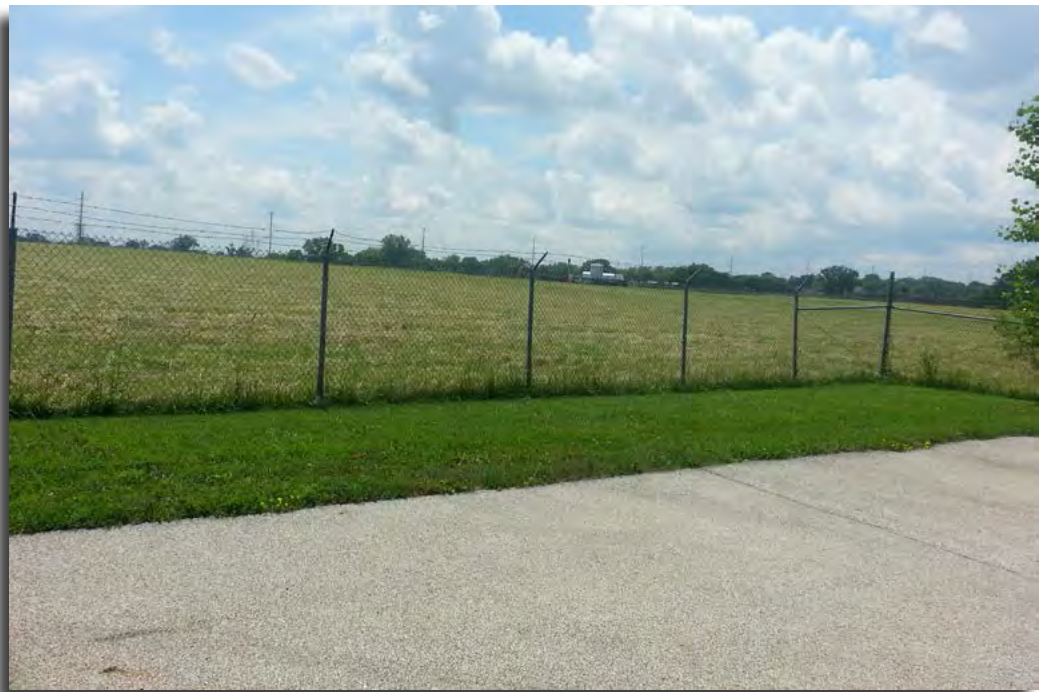
Photograph shows the fence installed around the Yeoman Creek Landfill.
