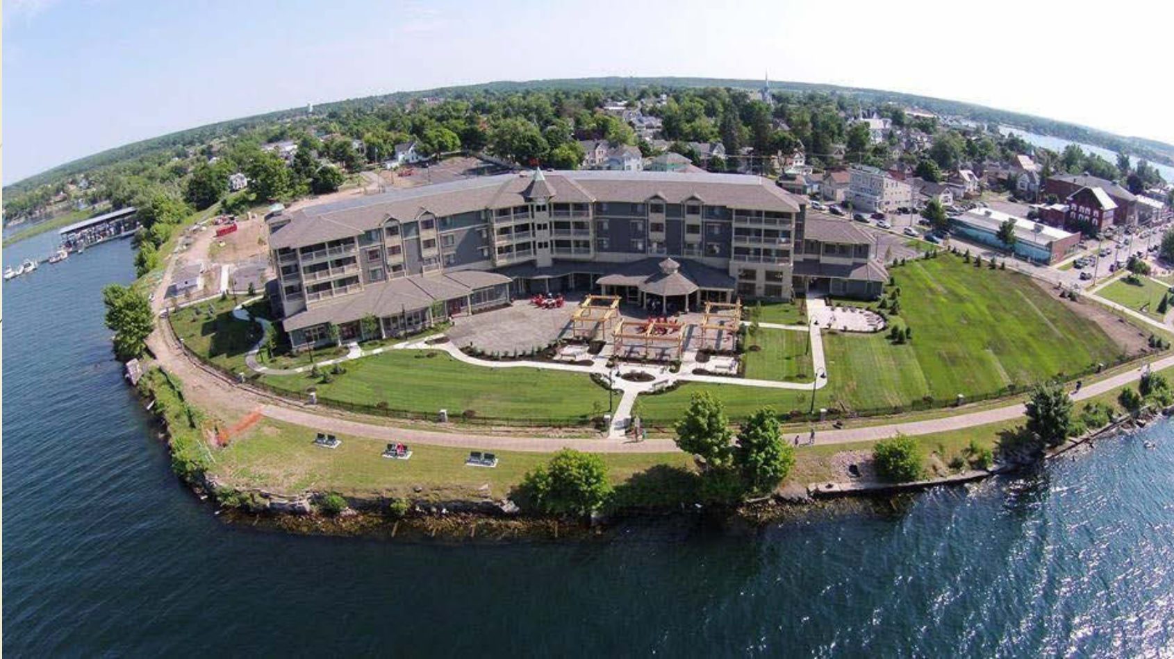
Former Superfund site in Clayton, New York along edge of St. Lawrence River Photo: 1000islandsharborhotel.com
