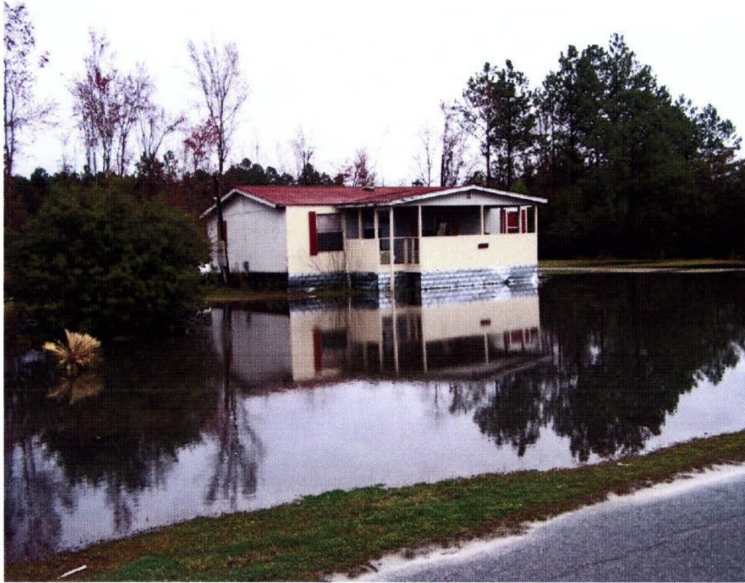
Robin Ln. near Hatton Still Rd. Intersection Inadequate size storm drain pipe backs up storm water in residents yards.
