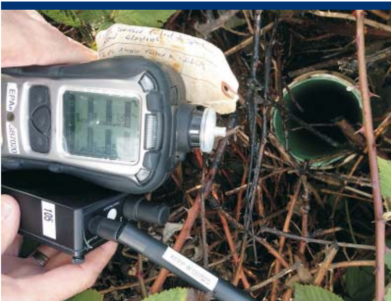
Photo 3 Monitoring effluent vapors from an open pipe on the west shoulder of Force Ave. The City of Portland later determined that it was related to the sewer and had been damaged.
