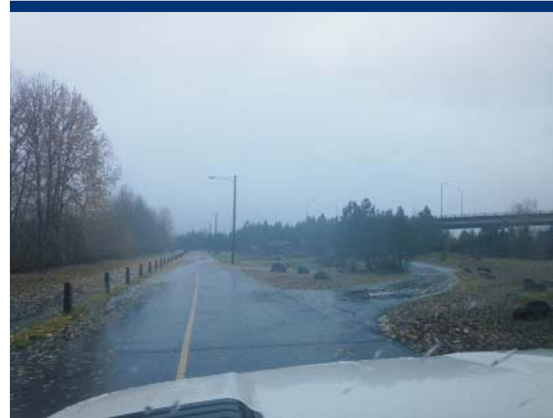
Photo 24 Mobile air monitoring west of Suttle Rd at Smith and Bybee Wetland Natural Area on a public access road. Direction: Northwest Date: 12/11/15 Time: 15:08
