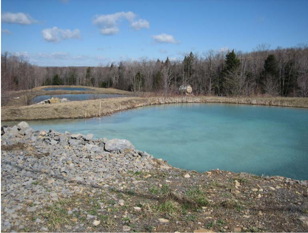
Figure 7-6. Photograph of the Three PBS Job #8 Settling Ponds
