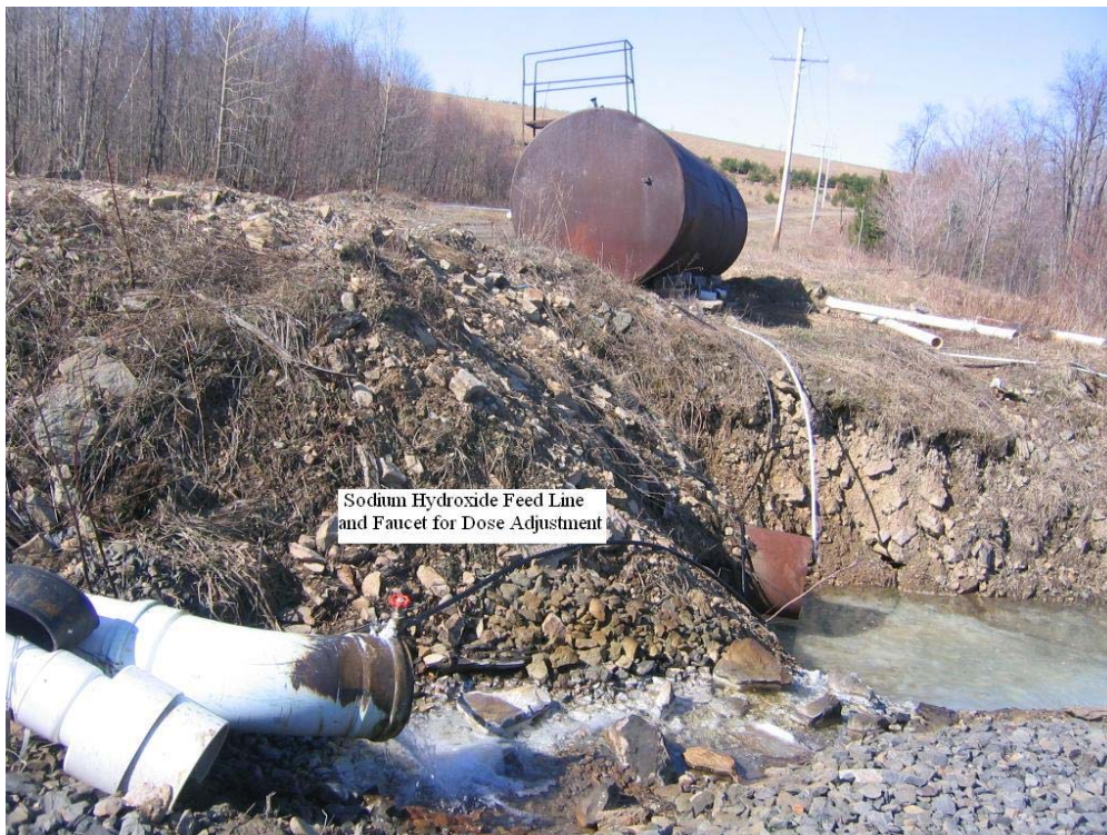
Figure 7-5. Photograph of Sodium Hydroxide Addition at PBS Job #8 Source: Site Visit Report Pennsylvania Coal Mine Acid Drainage Treatment Systems (ERG, 2006)
