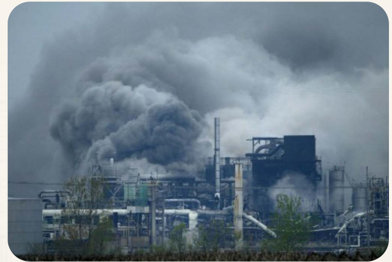
Formosa Plastics Plant Explosion, Illiopolis, Illinois, April 23, 2004 explosion. Photo: Kevin German/The State Journal-Register
