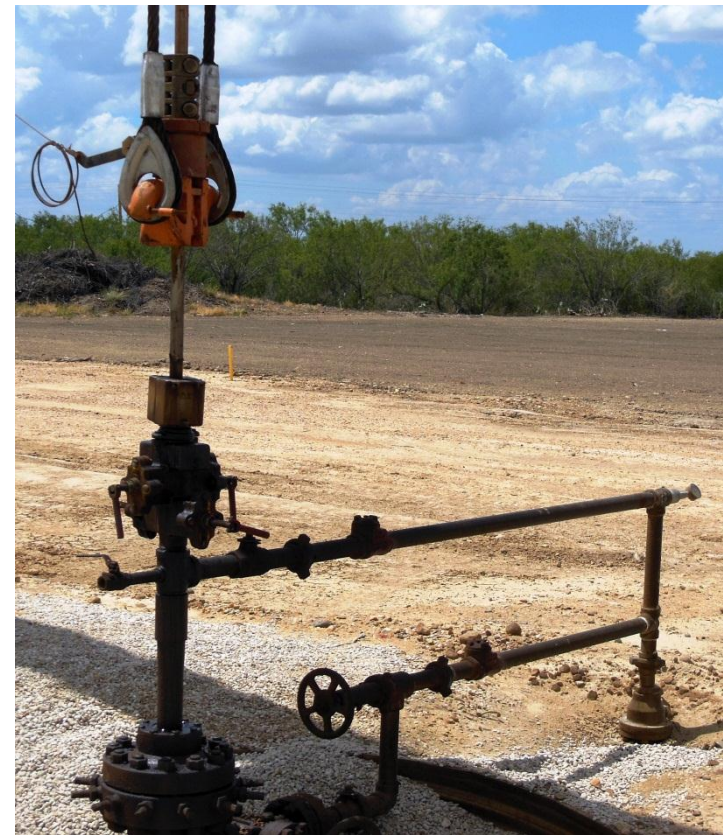
Wellhead with Pump Jack Unit
