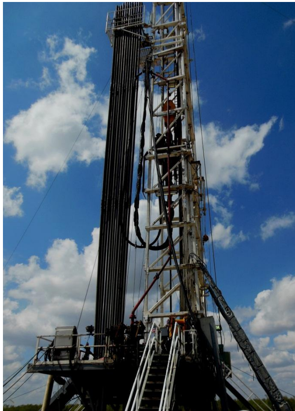
Drilling Rig (Typical)
