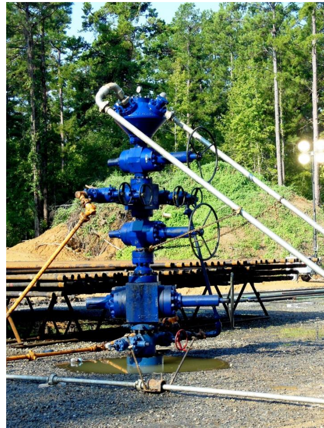
Wellhead Rigged for Fracking
