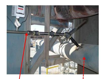
Engine air intake duct
